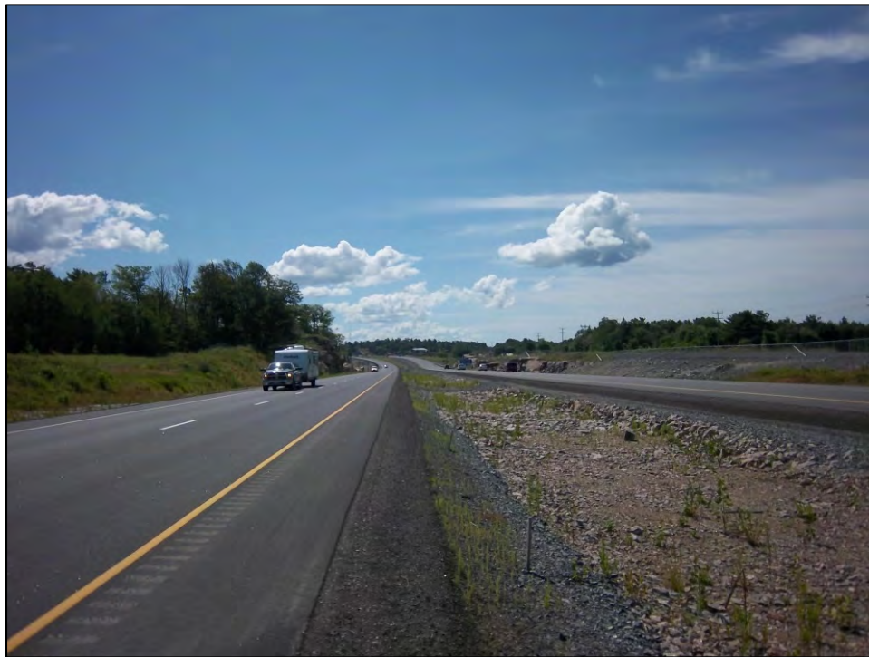
Example of a Four-Laned Section of Highway 11/17
