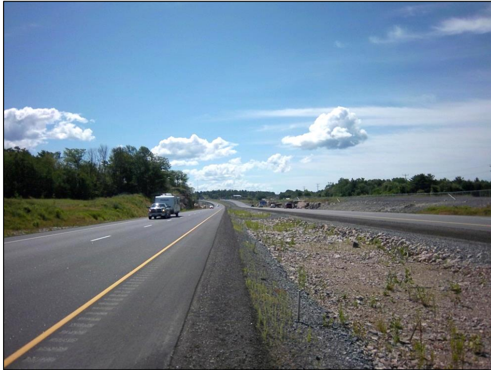
Example of a Four-Laned Section of Highway 11/17
